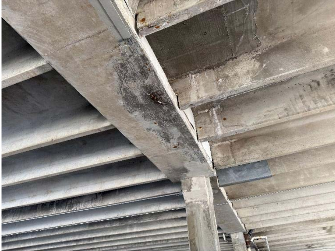
Concrete Degradation
